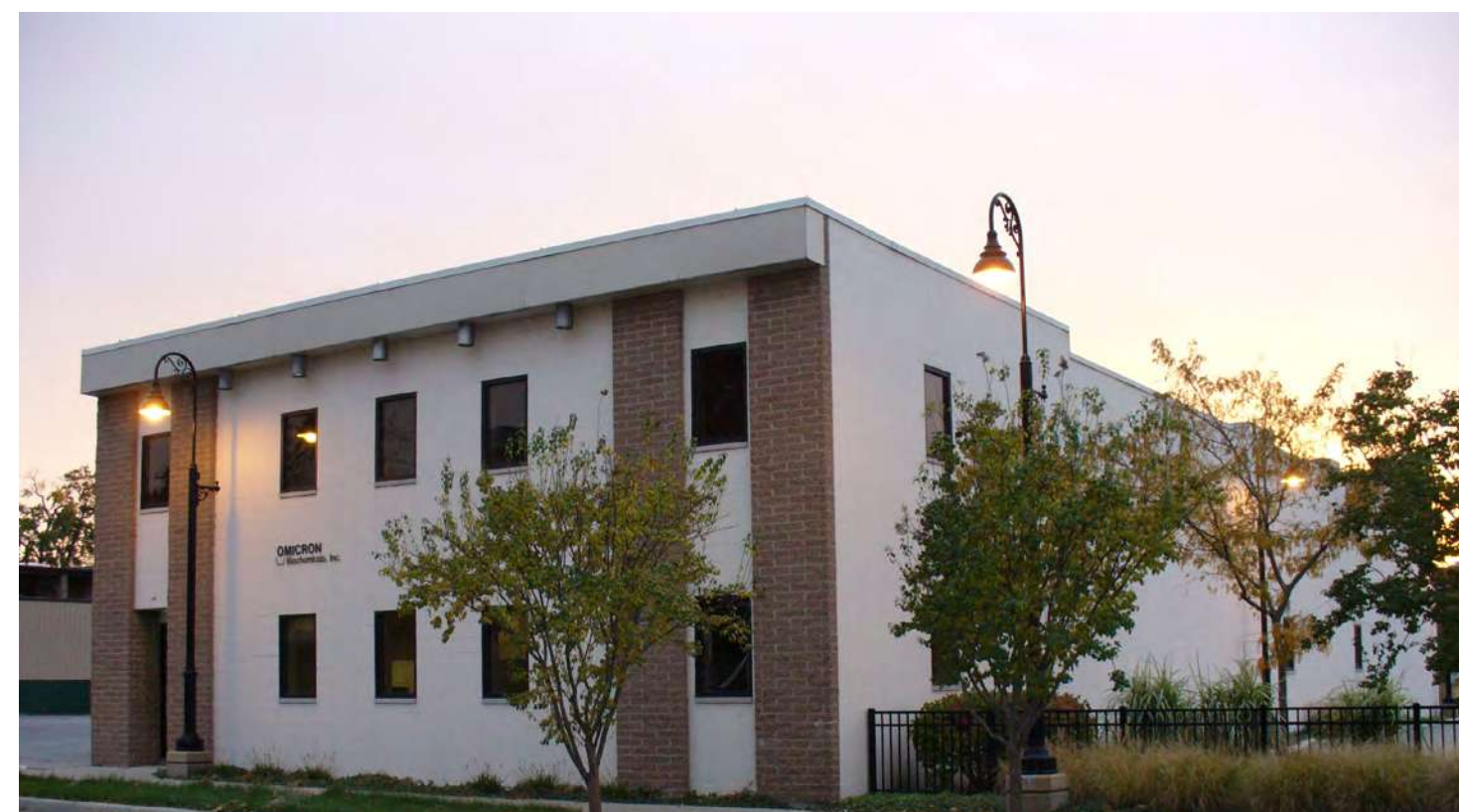
The Omicron R&D Facility in South Bend, Indiana
